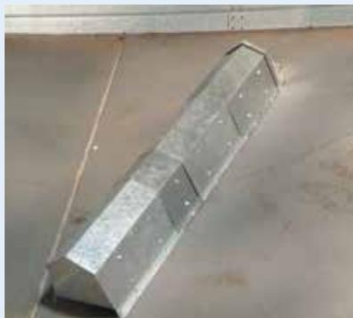
**Ducts lined up:** Aeration, especially aeration drying requires uniform airflow through the grain bulk. When retrofitting fans, ensure adequate size ducting is installed almost the full length of the silo cone. Where multiple fans are fitted, space them around the cone opposite each other.
