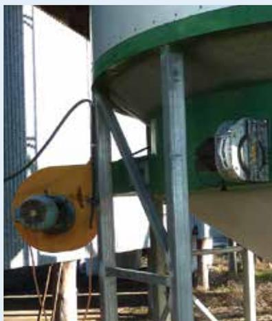
**Fans for the job:** This Kotzur drying silo is built with a high-airflow drying fan powered by a three phase, 7.5kW motor. The silo has been retrofitted with a small fan powered by a 0.37kW motor to provide aeration cooling after drying. To learn how to measure airflow read *Performance testing aeration systems fact sheet* by GRDC. <http://storedgrain.com.au/testing-aeration/>
