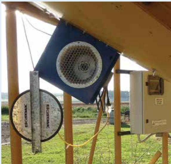
**Retro your silo:** This silo has been retro fitted with two fans opposite each other, powered by 1.5kW motors for aeration drying. The original pair of lower performance fans remain in place for aeration cooling.
